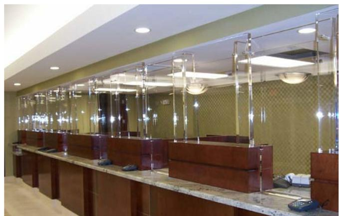
Plastic laminate with integrated Bullet Resistant Barrier.
