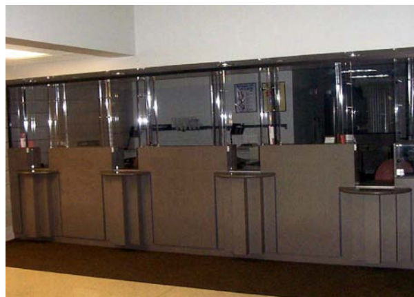
Plastic laminate – deco front accents with solid surface counter-tops & integrated bullet resistant barrier.
