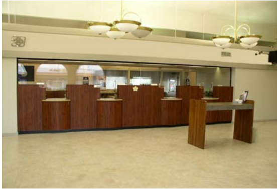
Plastic laminate – rounded fronts with solid surface counter-tops and integrated bullet resistant barrier
