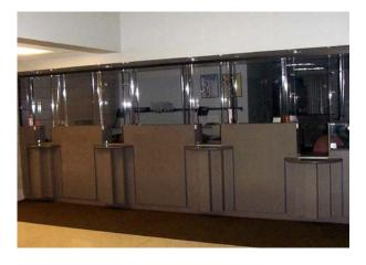
Plastic laminate – deco front accents with solid surface countertops & integrated bullet resistant barrier.
