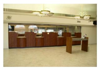
Plastic laminate – rounded fronts with Solid Surface countertops and integrated Bullet Resistant Barrier.
