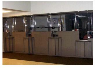
Plastic laminate – Deco front accents with solid surface countertops and integrated Bullet Resistant Barrier.
